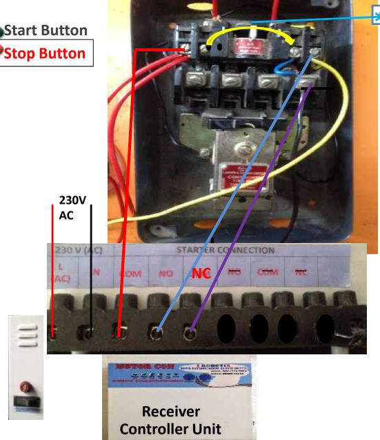
Remove jumper wire between start and stop button
